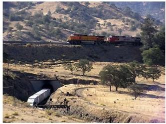
The head (above) is about to "bite the tail" coming out of the tunnel below. From top-of-rail above the tunnel to top-of-rail in the tunnel, trains gain or lose 77 feet while traversing the Tehachapi Loop.
